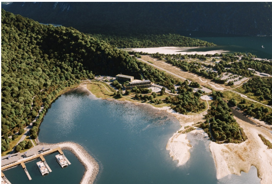
Figure 21: Milford Sound Piopiotahi 3D model of visitor hub & accommodation and staff accommodation buildings
