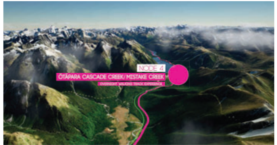
Figure 24: Aerial view of Node 4 - Ōtāpara Cascade Creek / Mistake Creek overnight walking track experience
