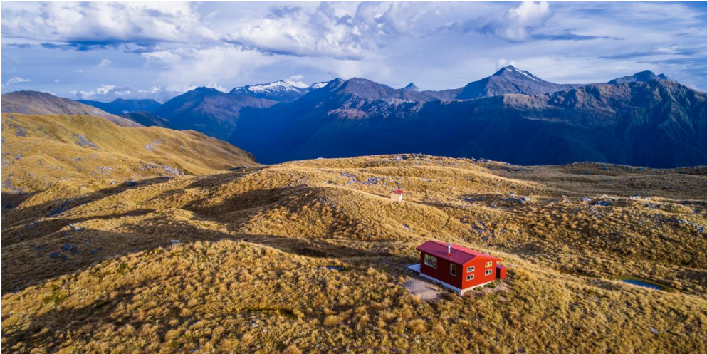
Figure 12. Helicopter view of Mataketake Hut, showing the vista. (Photo: Backcountry Trust).
